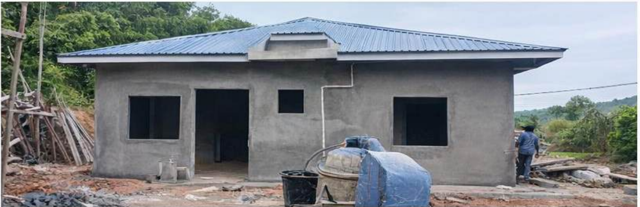
Plastering & roofing stage
