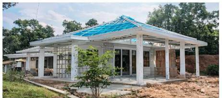
House near completion
