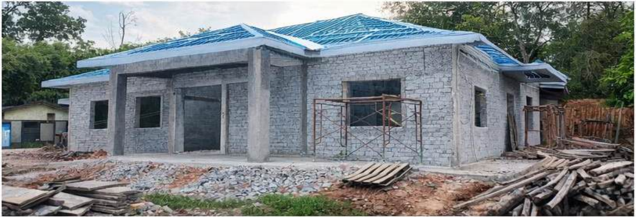
Structure & brickwork stage
