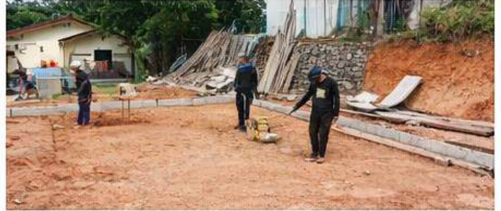
Marking and excavation
